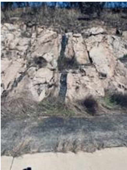
Figure 19: Two thrust faults evident in this road cutting
